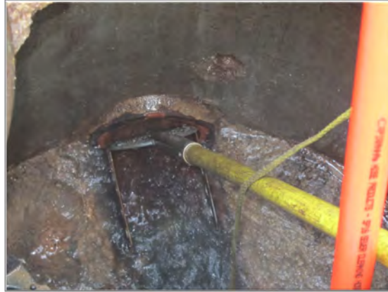
Photo 7-5. Tipping a Debris Trap to Relieve Backed Up Water
