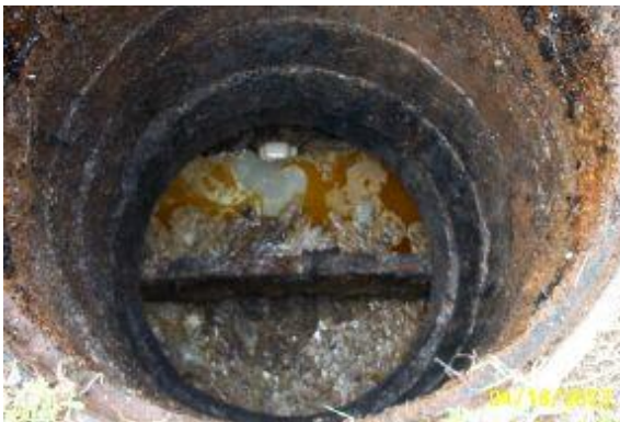
No outlet T, even with additional baffle, FOG can be Discharged if there is no outlet T attached
