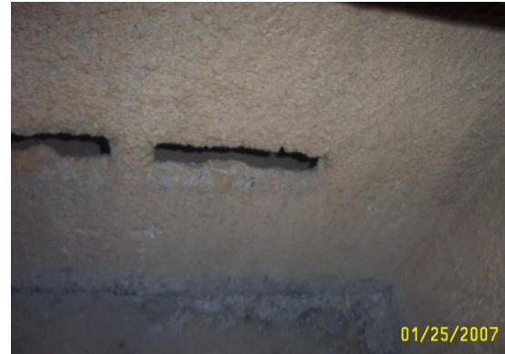
Slit style baffle walls, are not as efficient as the single hole baffle wall design
