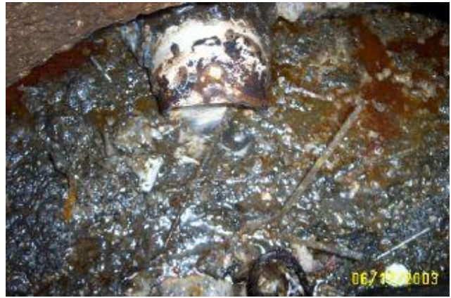
No Inlet T! Also, straws, stirrers, trash
