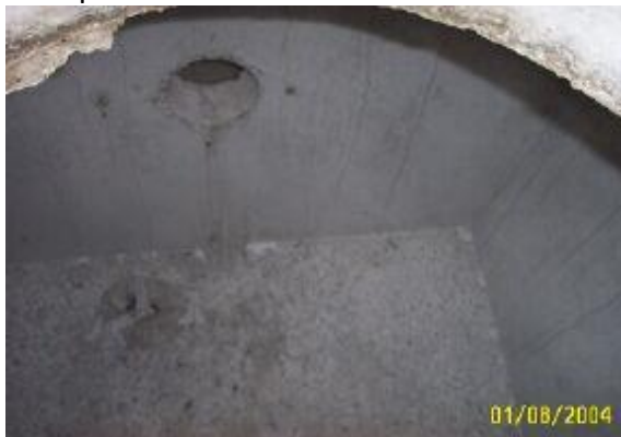
Single hole in baffle wall
