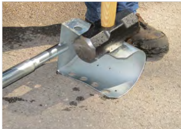
Photo 7-4. Using a Sledge Hammer to Slightly Modify a Debris Trap
