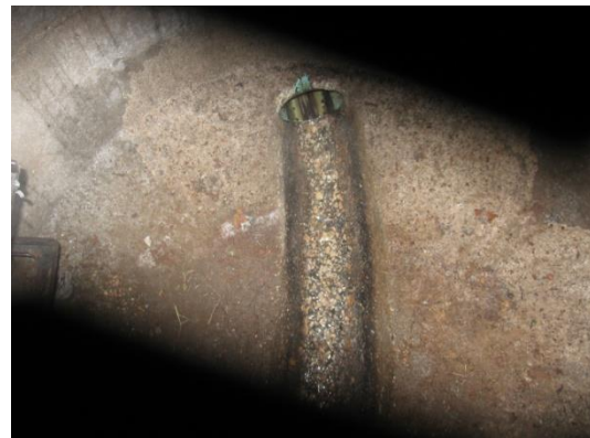
Concrete deterioration in invert below coffee shop
