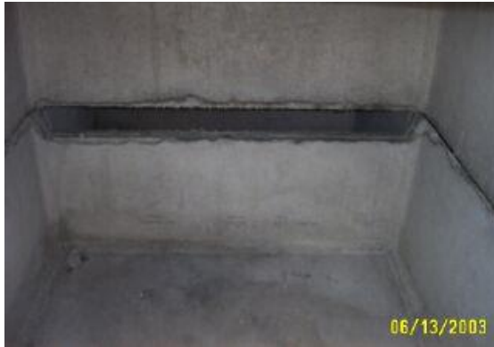
Slit style baffle walls, are not as efficient as the single hole baffle wall design
