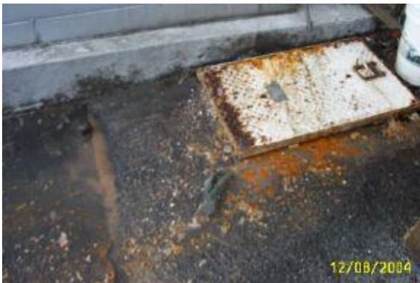
Outside floor trap that has overflowed. Undersized for this FSE, need large grease trap. Inspector should check downstream sewer lines and issue a NCN to the FSE. Also, the inspector should contact the Health Dept and Stormwater personnel.
