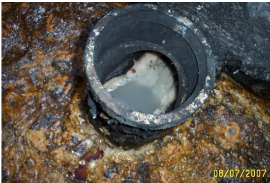
Examples of FOG in outlet T that indicate FOG discharge to sewer system
