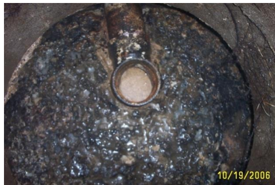
Examples of FOG in outlet T that indicate FOG discharge to sewer system
