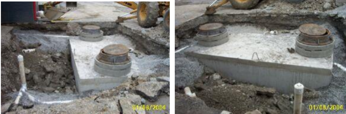
Typical Grease Trap installation with two manhole access
