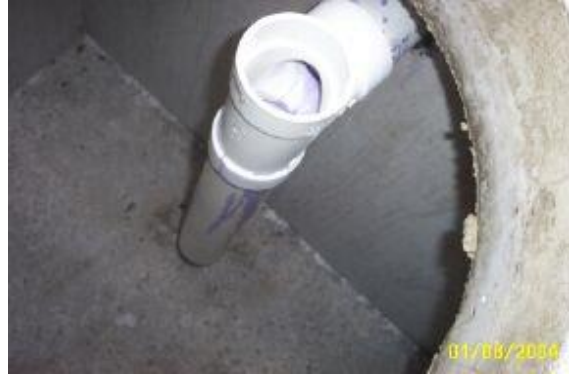
Example of properly installed schedule 40 PVC Outlet T
