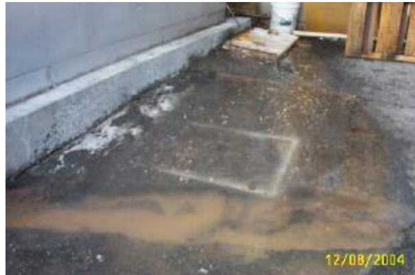
Outside floor trap that has overflowed. Undersized for this FSE, need large grease trap. Inspector should check downstream sewer lines and issue a NCN to the FSE. Also, the inspector should contact the Health Dept and Stormwater personnel.
