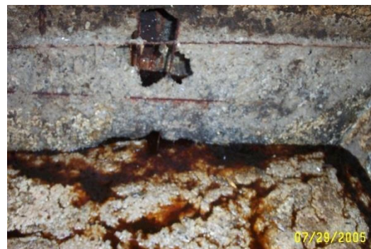
Concrete deterioration in invert below coffee shop
