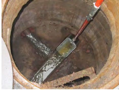
Photo 7-3. Debris Trap Placed in Manhole Channel
