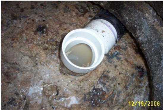
Example of clear water in outlet T (Good!)
